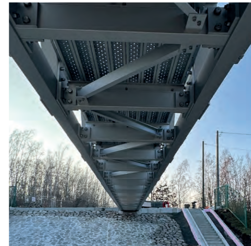
Truss bracing floor for greater stability
