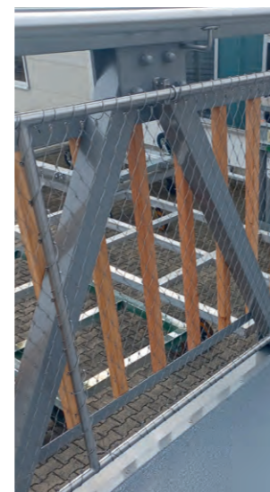
Railing infill with stainless steel wire mesh.
