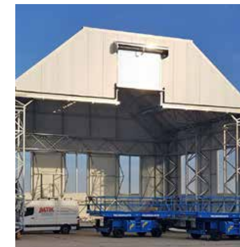
Roller shutter gate is located on top of the front wall.
